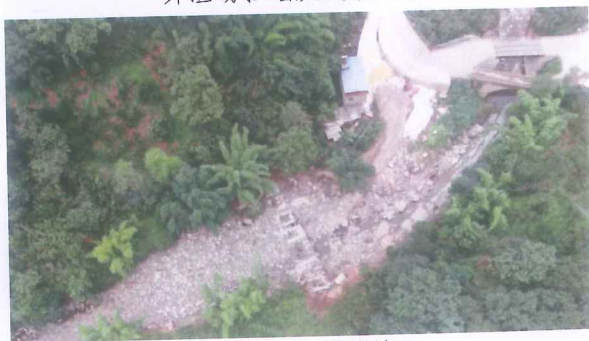
弃渣场底部挡墙
