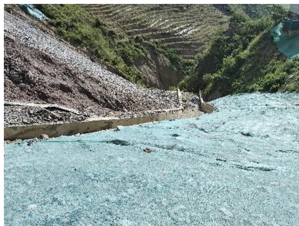
隧道临时苫盖
