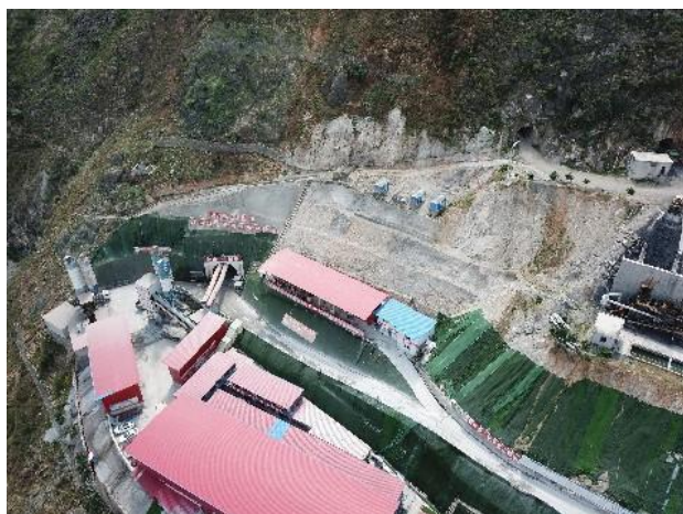
隧道临时苫盖
