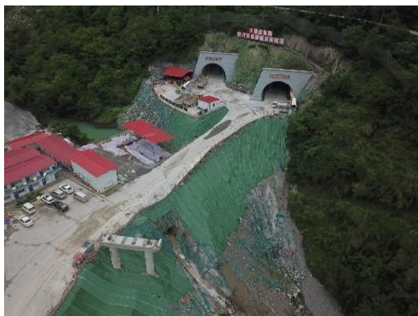
隧道临时苫盖
