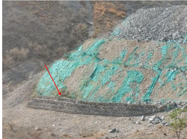
临时转运场铅丝石笼
