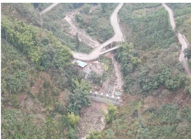
弃渣场底部挡墙
