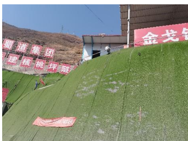
边坡临时苫盖
