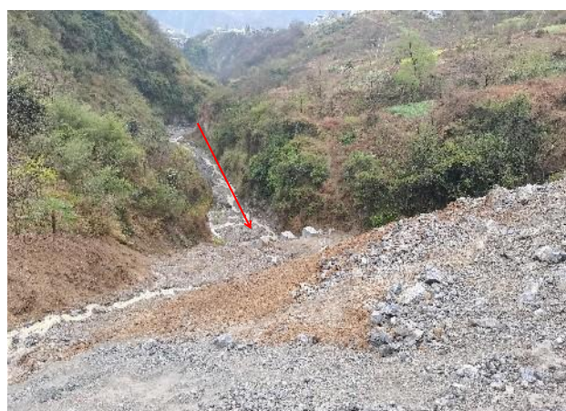
弃渣场底部挡墙
