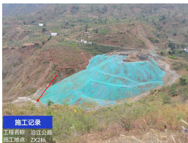
弃渣场底部挡墙
