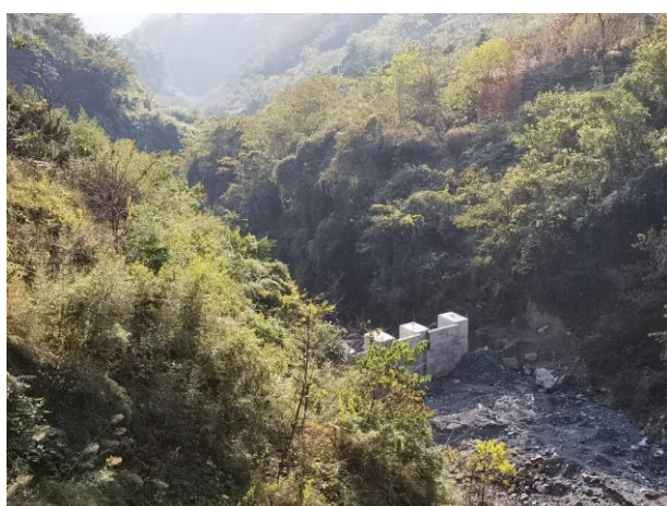
弃渣场底部挡墙
